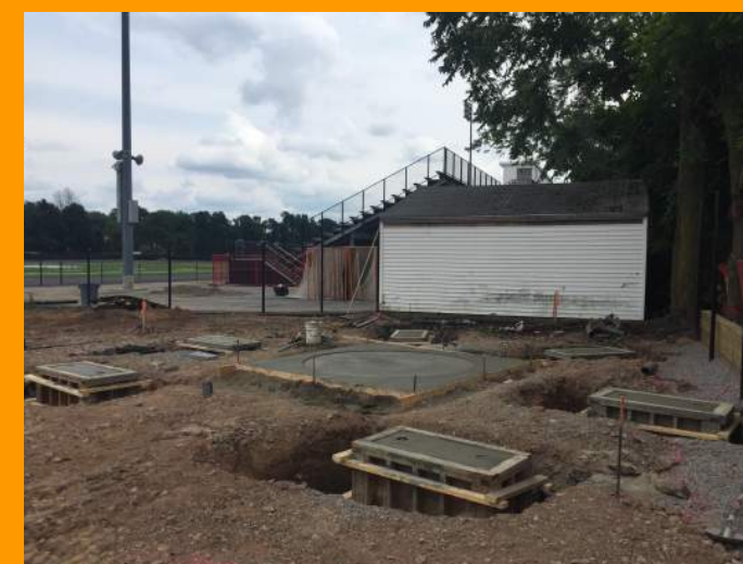
New Discus Throwing Pad and Foundations
