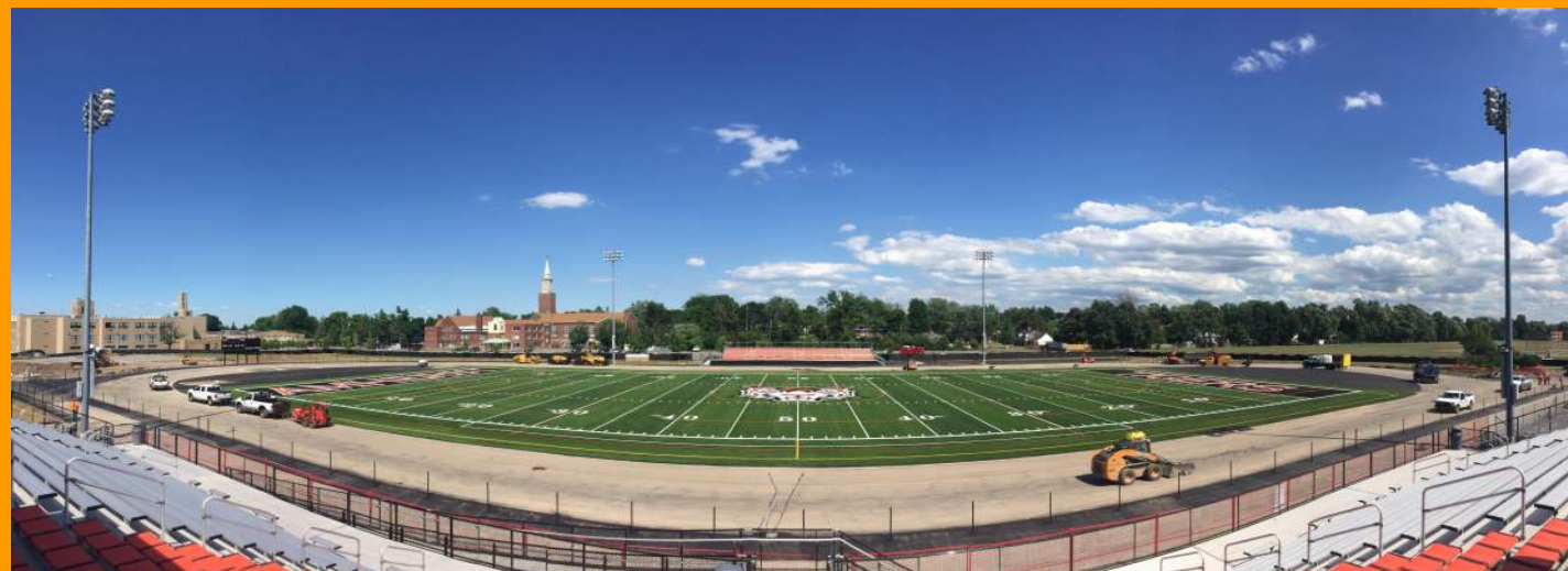
Completion of New Turf Field - Preparation of Track for Asphalt
