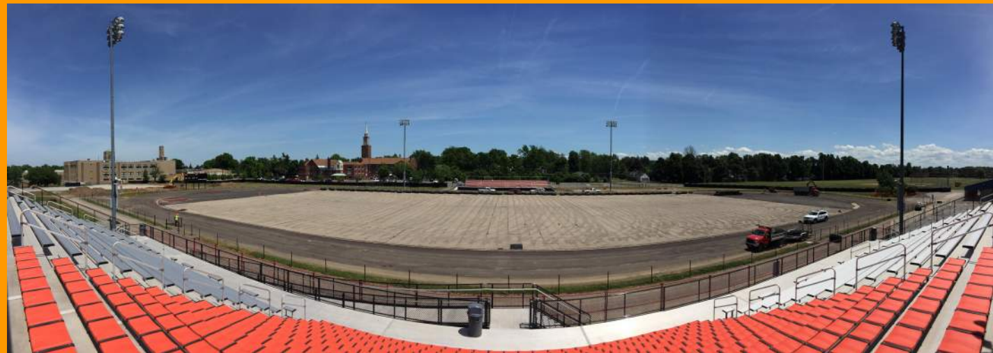
Existing Turf Field Removed - Installation of Stone Dust
