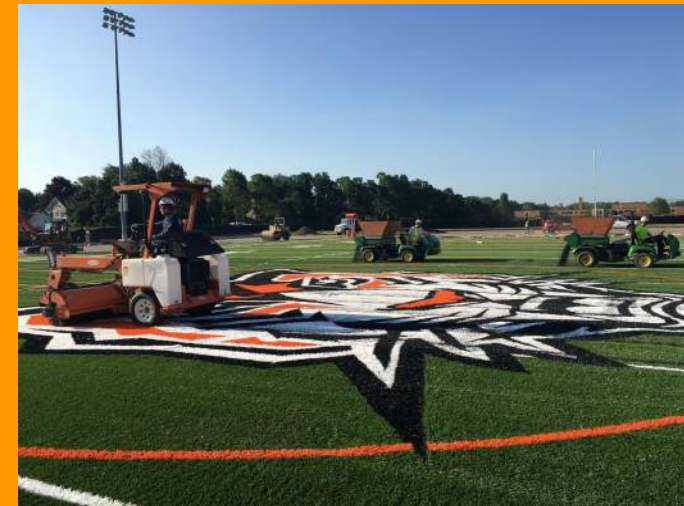
Installation of Rubber Infill and Grooming
