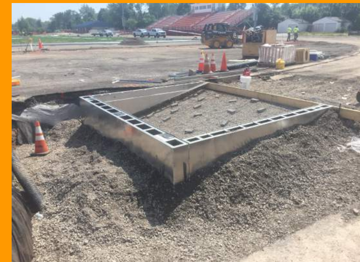
New Steeple Chase Foundations and Pit
