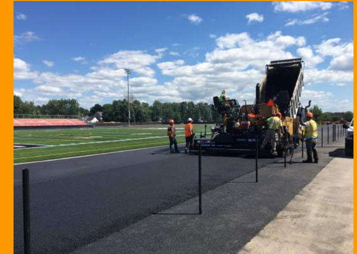
New Asphalt Pavement at Track
