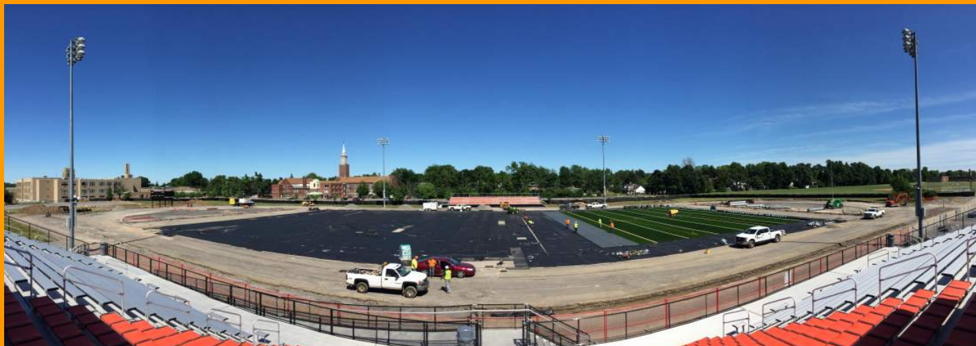
Installation of Rubber Shock Pad - Installation of New Turf and Inlays
