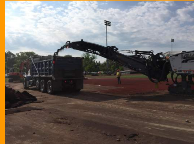
Milling of Existing Track and Asphalt Layers
