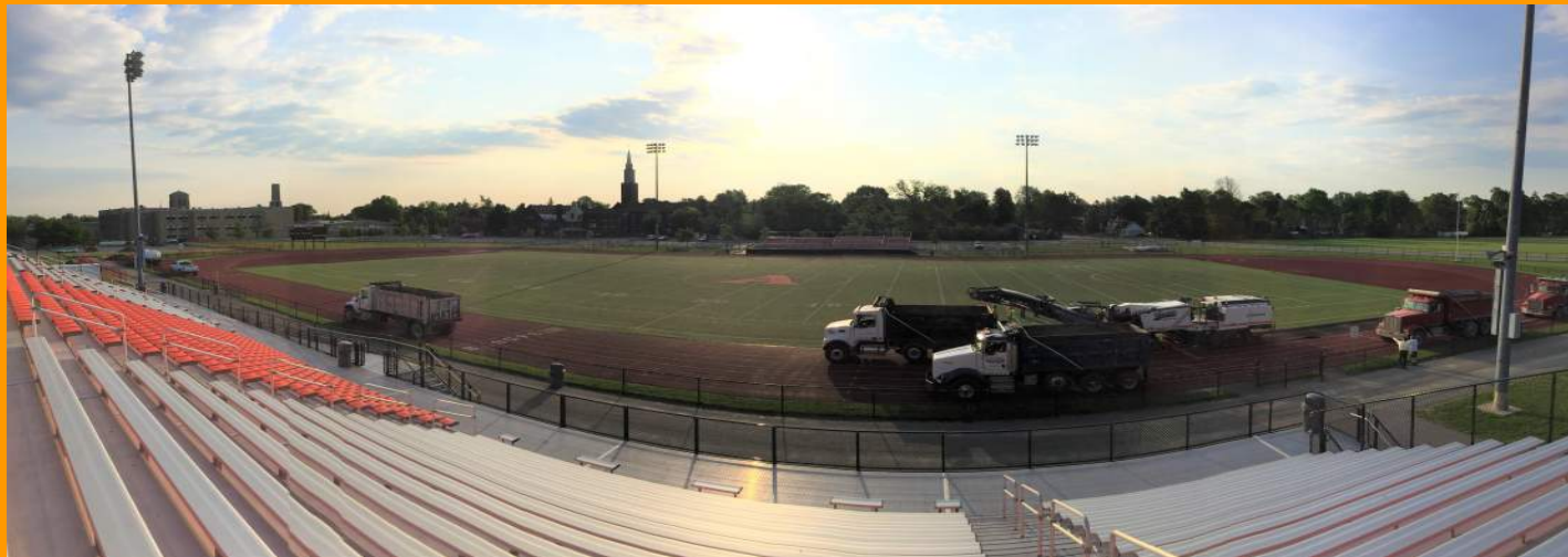
Original Turf Field - Original Track Removal
