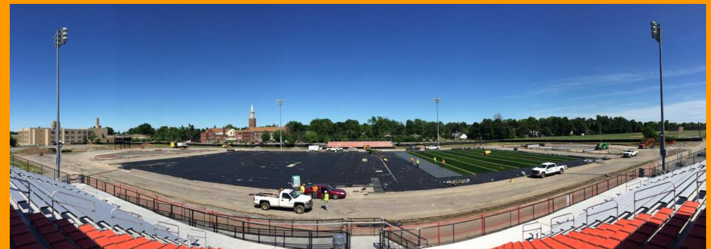
New Shock Pad and Turf Field Inlays Installation
