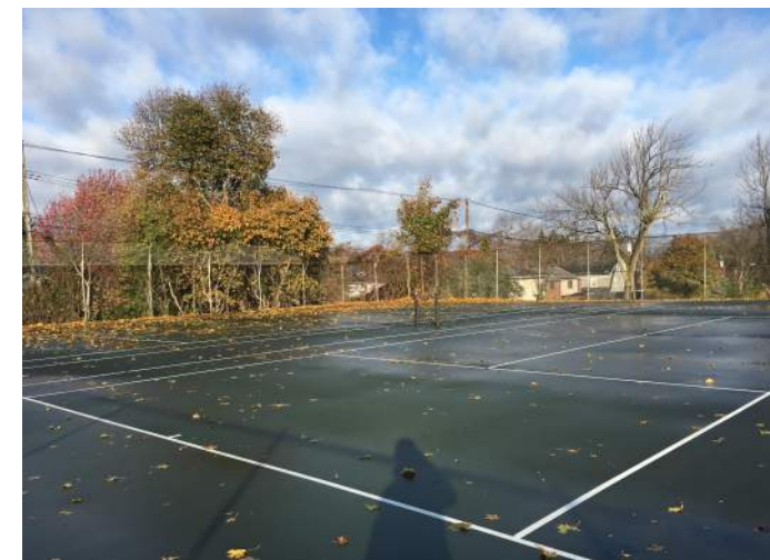
Original Tennis Courts and Fencing
