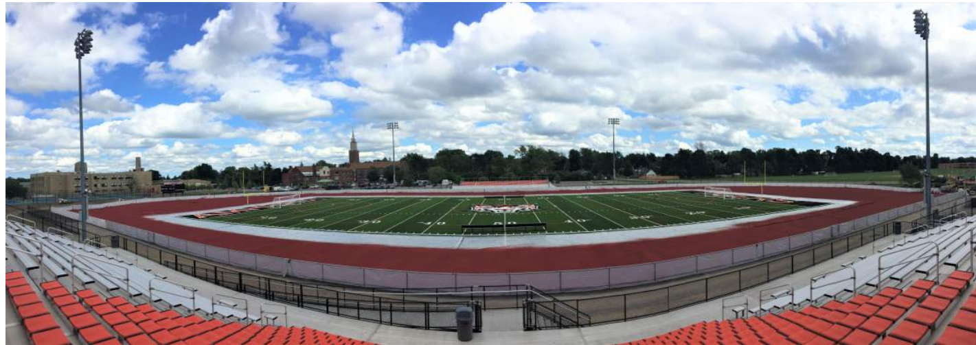
New Rubber Track Surface Installation
