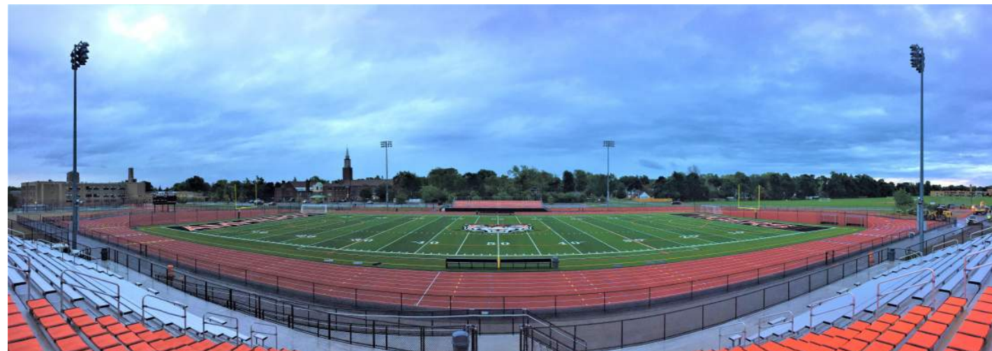
New Track and Field Completed
