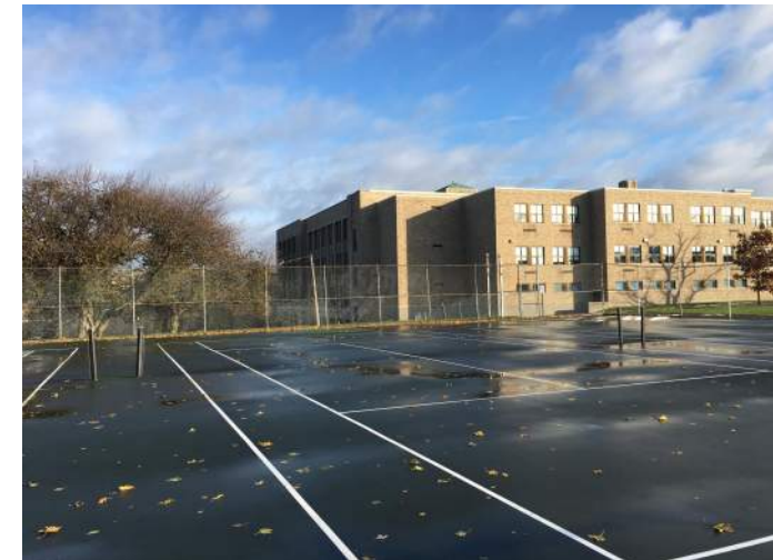
Original Tennis Courts and Fencing
