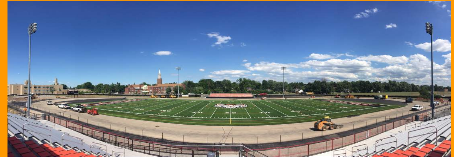
New Turf Field Installation - New Asphalt Top Install
